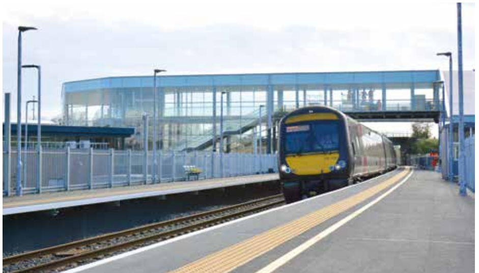
Greenfield to green station in six years: CrossCountry's No 170101 passes the future site of Worcestershire Parkway's Birmingham-bound platform on 25 May 2013 with a Cardiff to Nottingham service (top) and No 170102 (above) on the same service on 29 October 2019 as the pre-opening finishing touches are put to the station. The North Cotswold line between Worcester and Paddington crosses from right to left on the overbridge. Steve Widdowson
