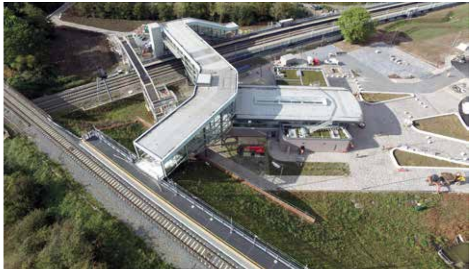
New station: Worcestershire Parkway approaching completion in October 2019. The North Cotswold line platform is at the foot of the picture, with the Paddington direction to the right. The Bristol to Birmingham line platforms run left to right. Courtesy Worcestershire County Council
